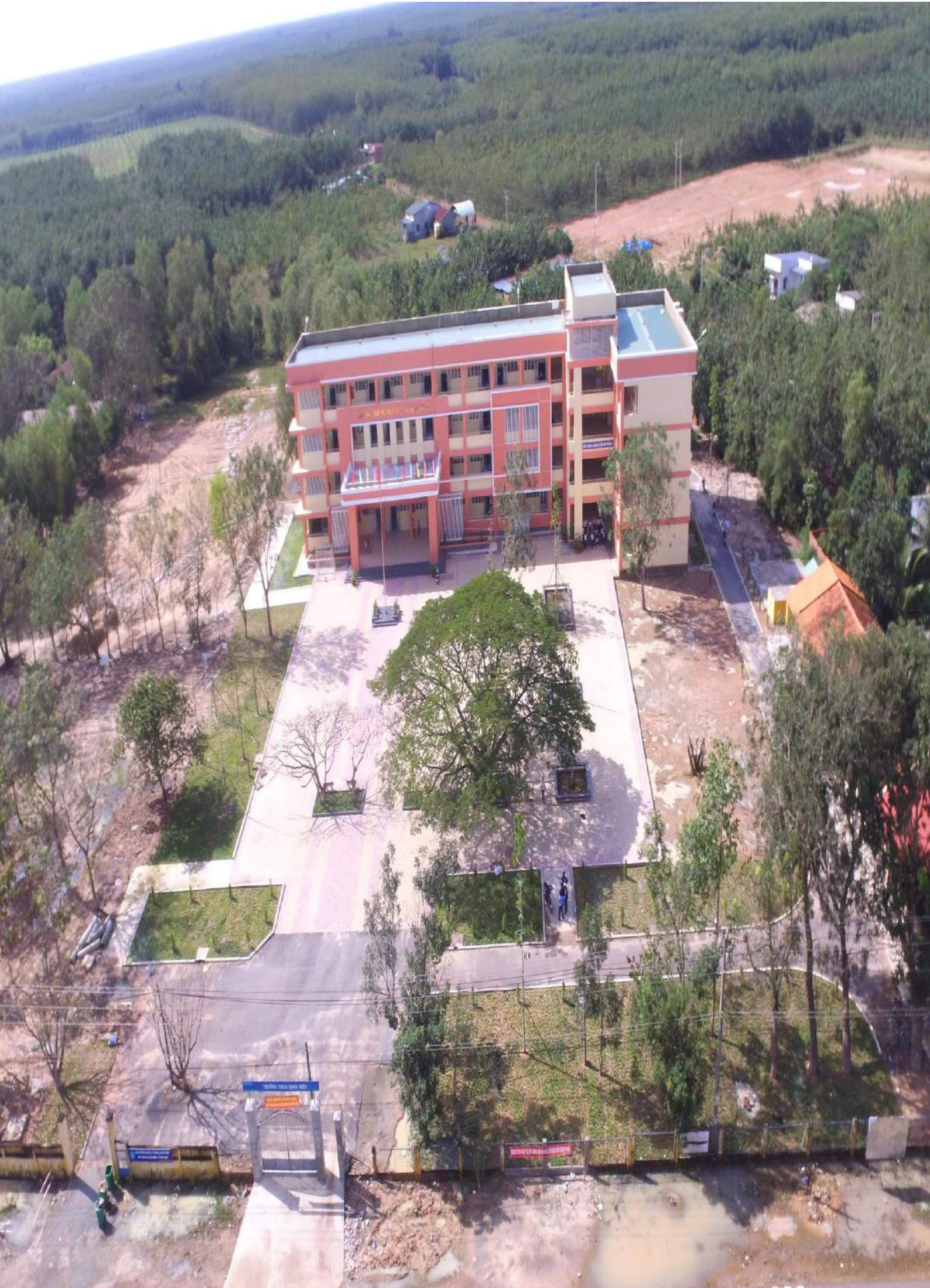
SECONDARY SCHOOL PROJECT CONSTRUCTED BY C32
