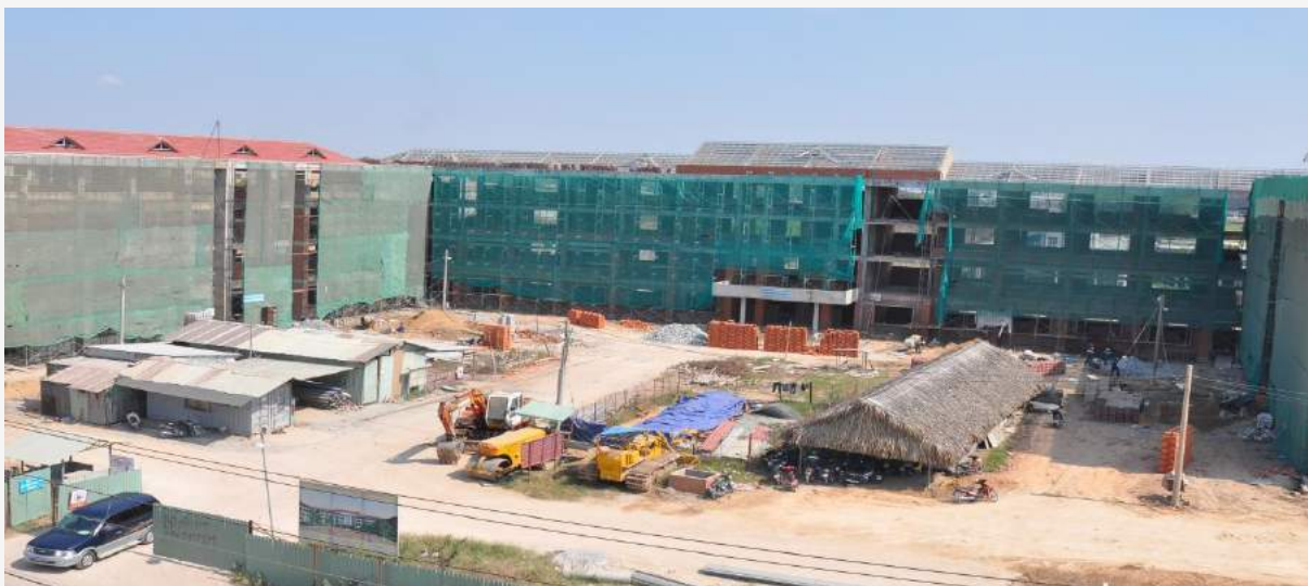
THUAN GIAO SECONDARY SCHOOL_C32 HAS BEEN CONSTRUCTING
