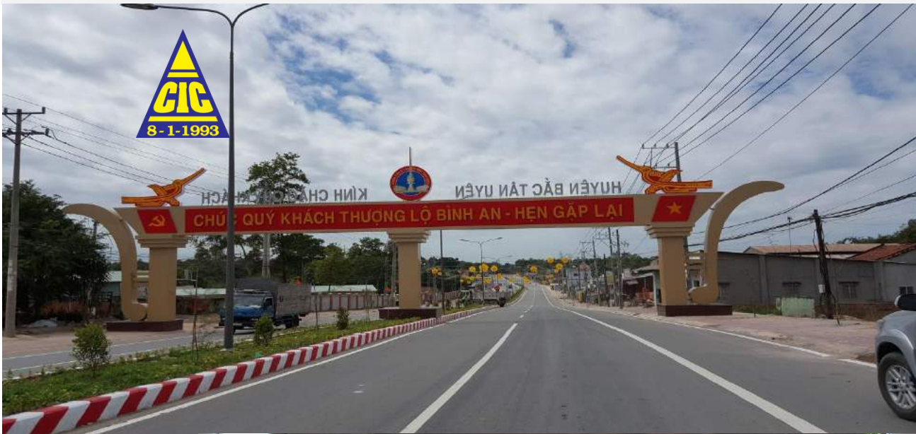
MUOI MUON STREET CONSTRUCTED BY C32
