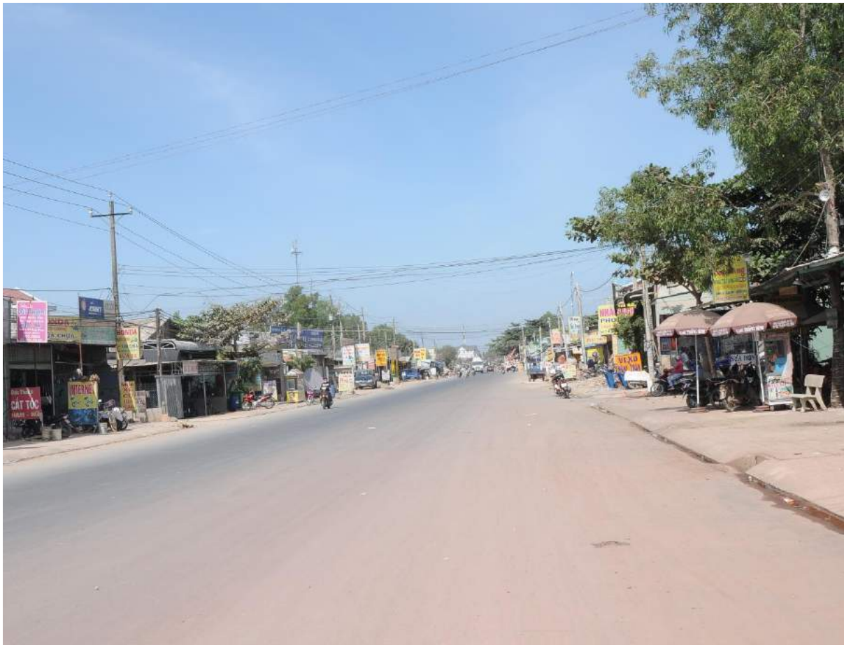
LE HONG PHONG STREET PROJECT CONSTRUCTED BY C32
